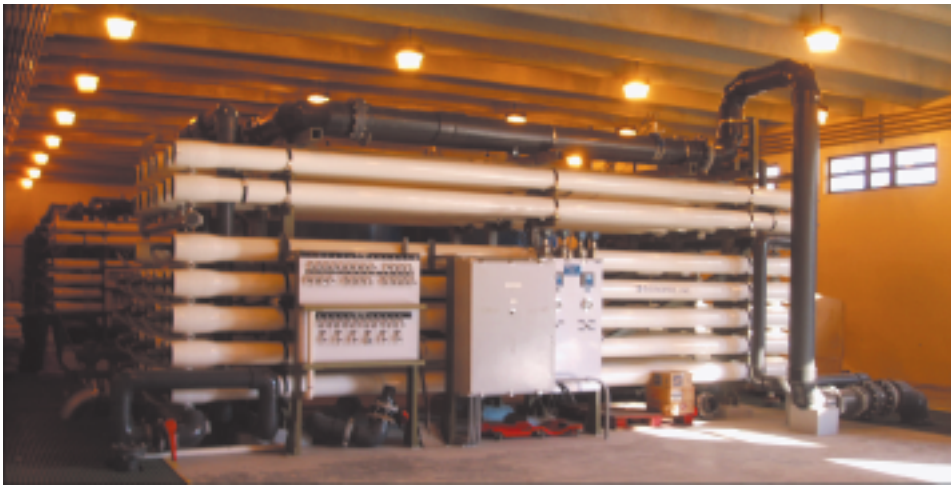
St. Lucie West District RO Water Treatment Plant: Two 1.7 MGD trains (two-stage system, 20:12 array configuration, seven elements per pressure vessel, side-port pressure vessels, interstage boost/energy recovery device.
